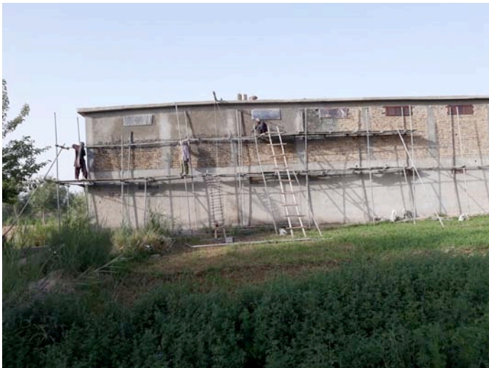
Plastering second floor classrooms
