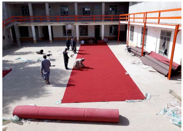
Cutting carpet in the courtyard
