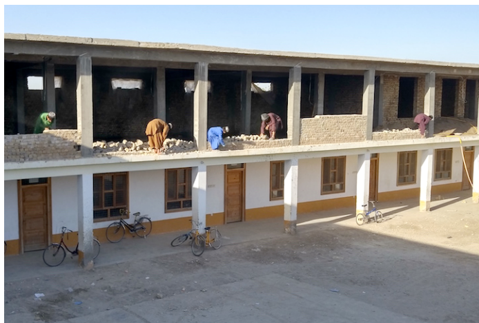
Second floor classrooms’ wall construction
