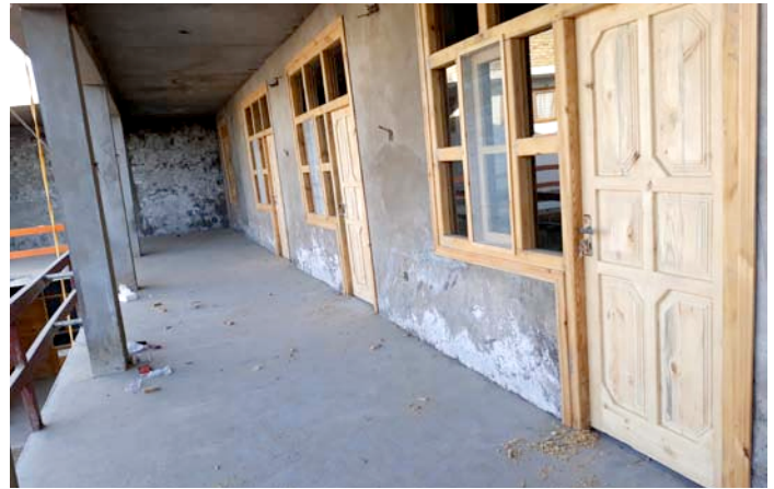
Doors and windows installation for second floor classrooms
